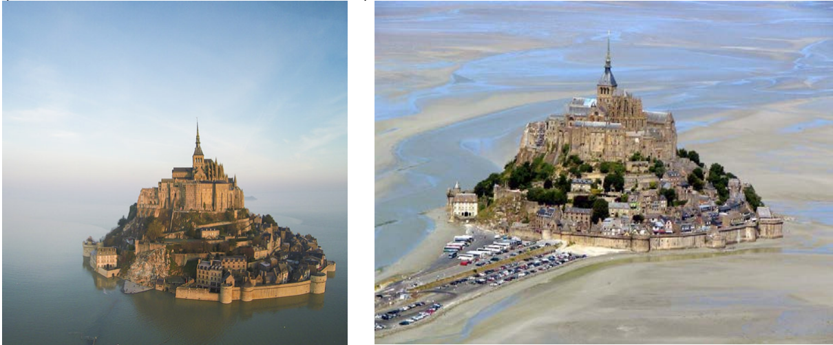
Figure D2: Low tide at Mont Saint-Michel, France, 2005, right ( http://www.ulm.it/hangar/mix/beltrutto/lemont/msm.htm ).
